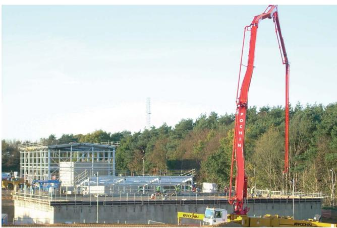
63 metre concrete pump pouring reservoir roof
