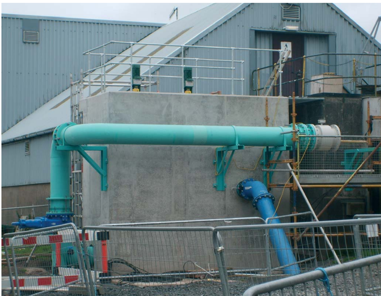
Corsehouse WTW Inlet works under construction
