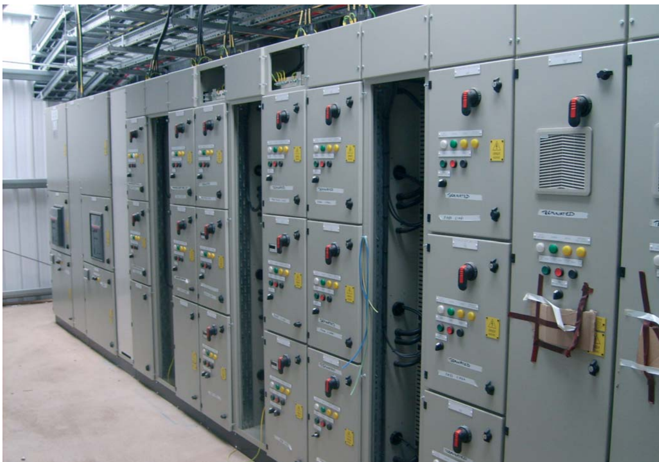
Corsehouse WTW MCC Room during installation
