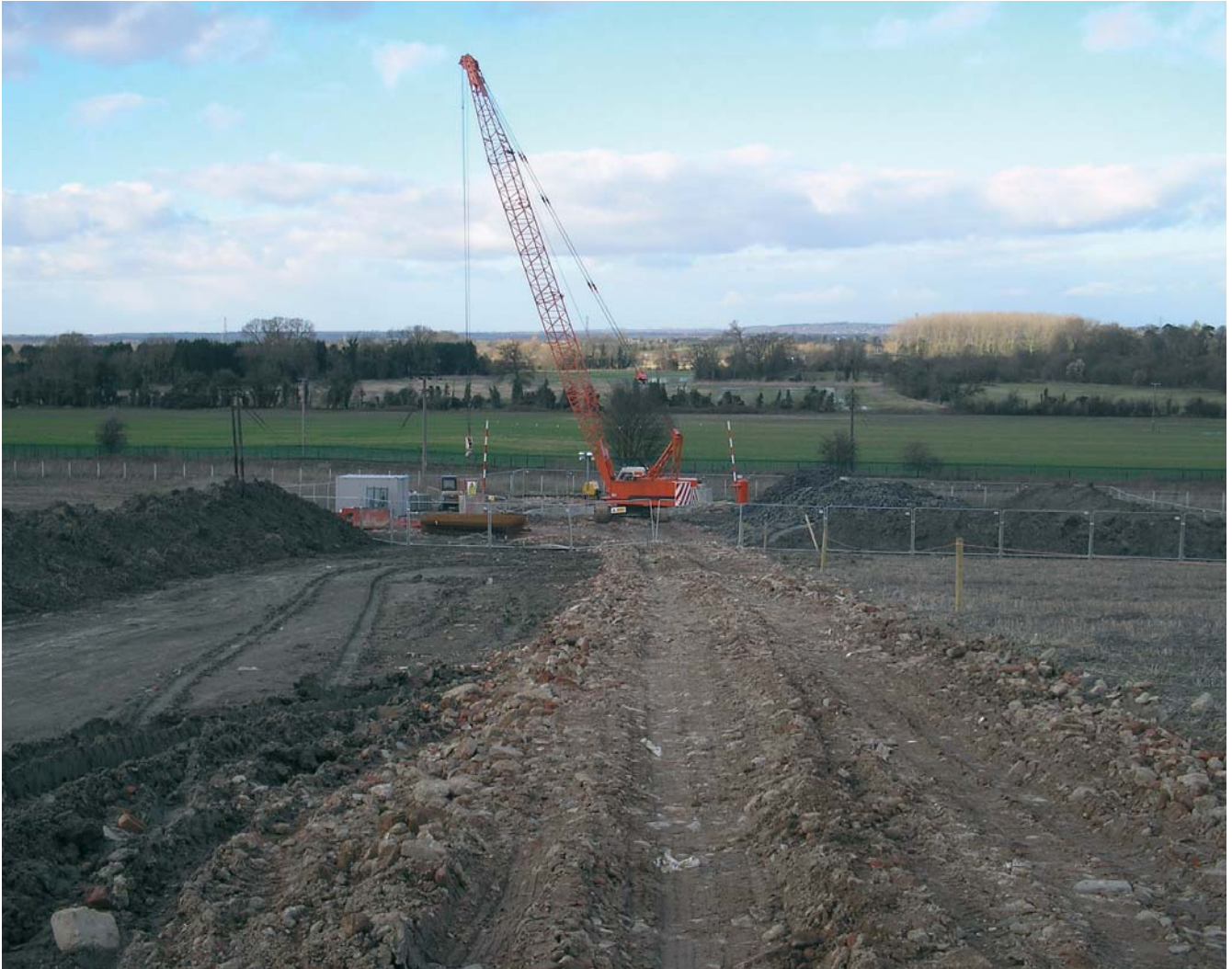
Steventon Rail Crossing - South Side Shaft Works
