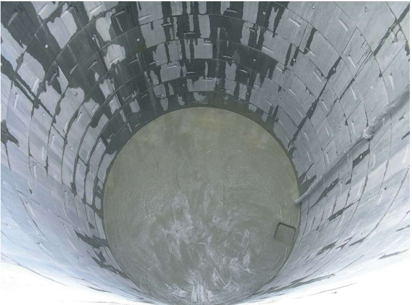
Steventon Rail Crossing - South Shaft - Interior prior to tunnelling
