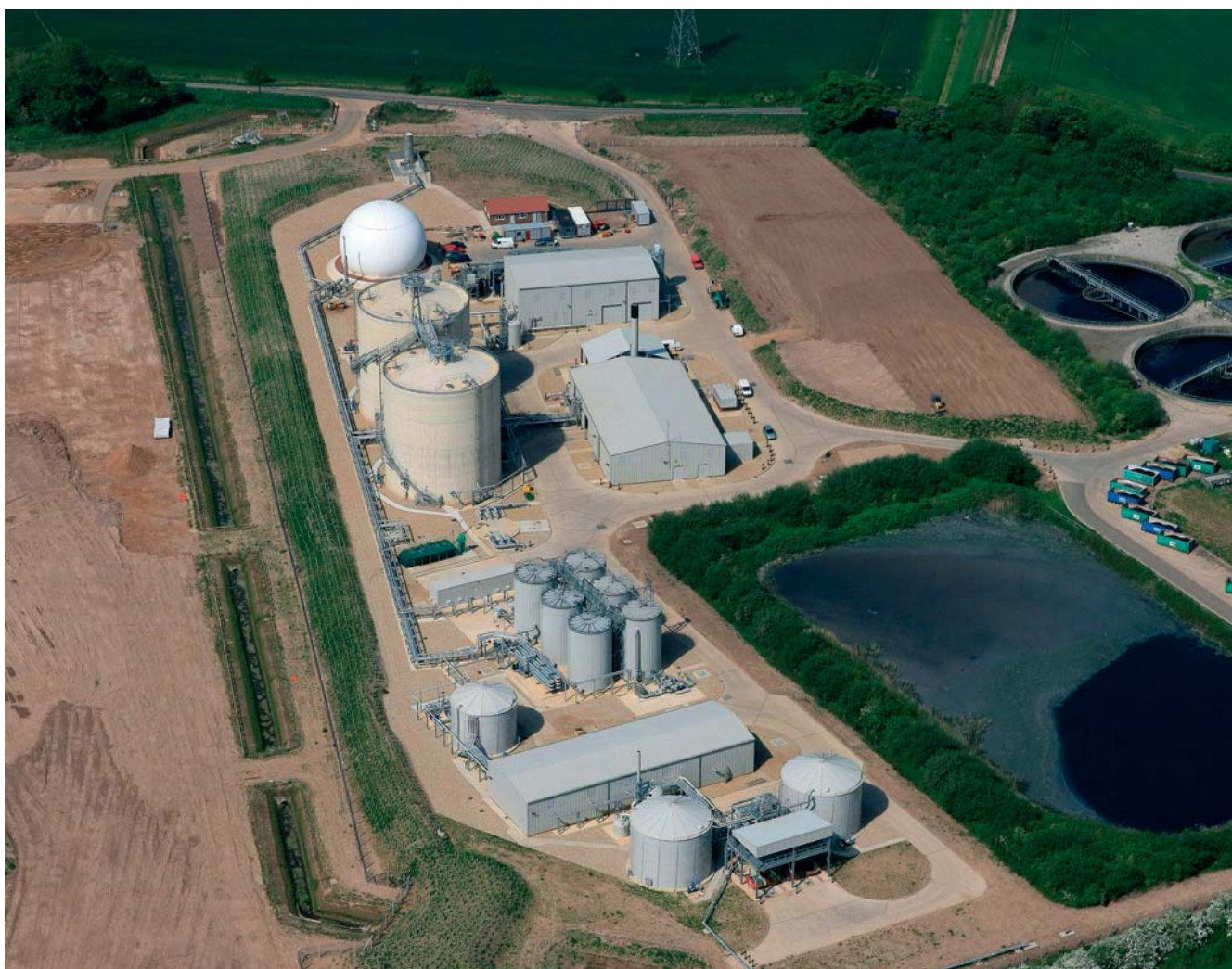
Kings Lynn Biosolids Treatment Centre
