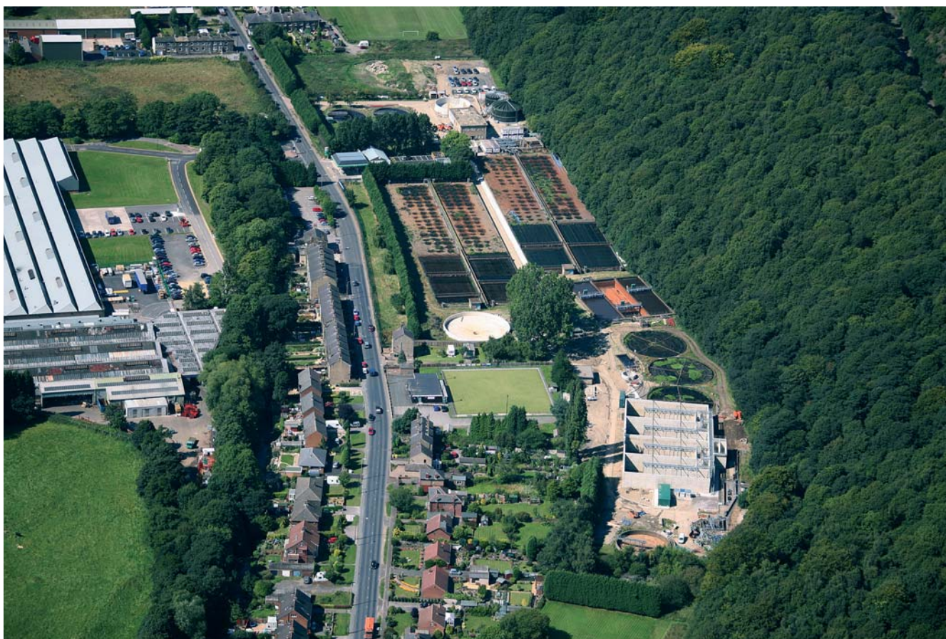
Aerial photograph of Neiley WwTW showing restricted site available for construction
