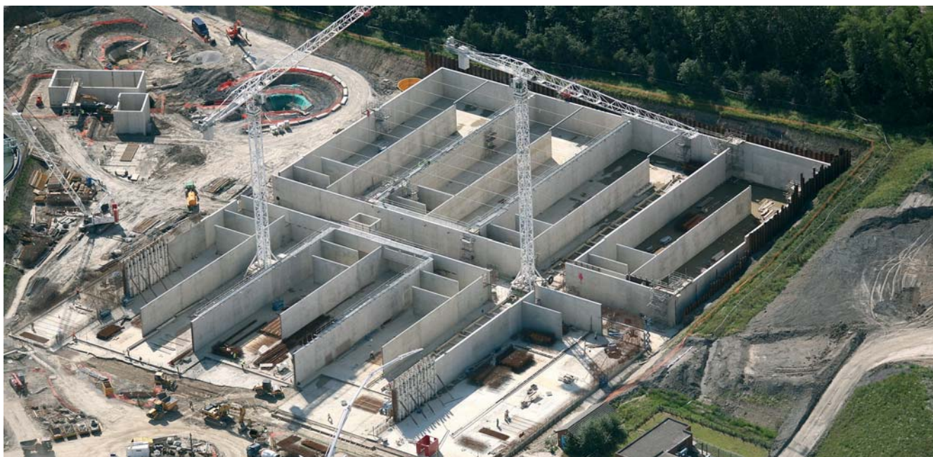
New Activated Sludge Plant under construction at Knothrop WwTW
