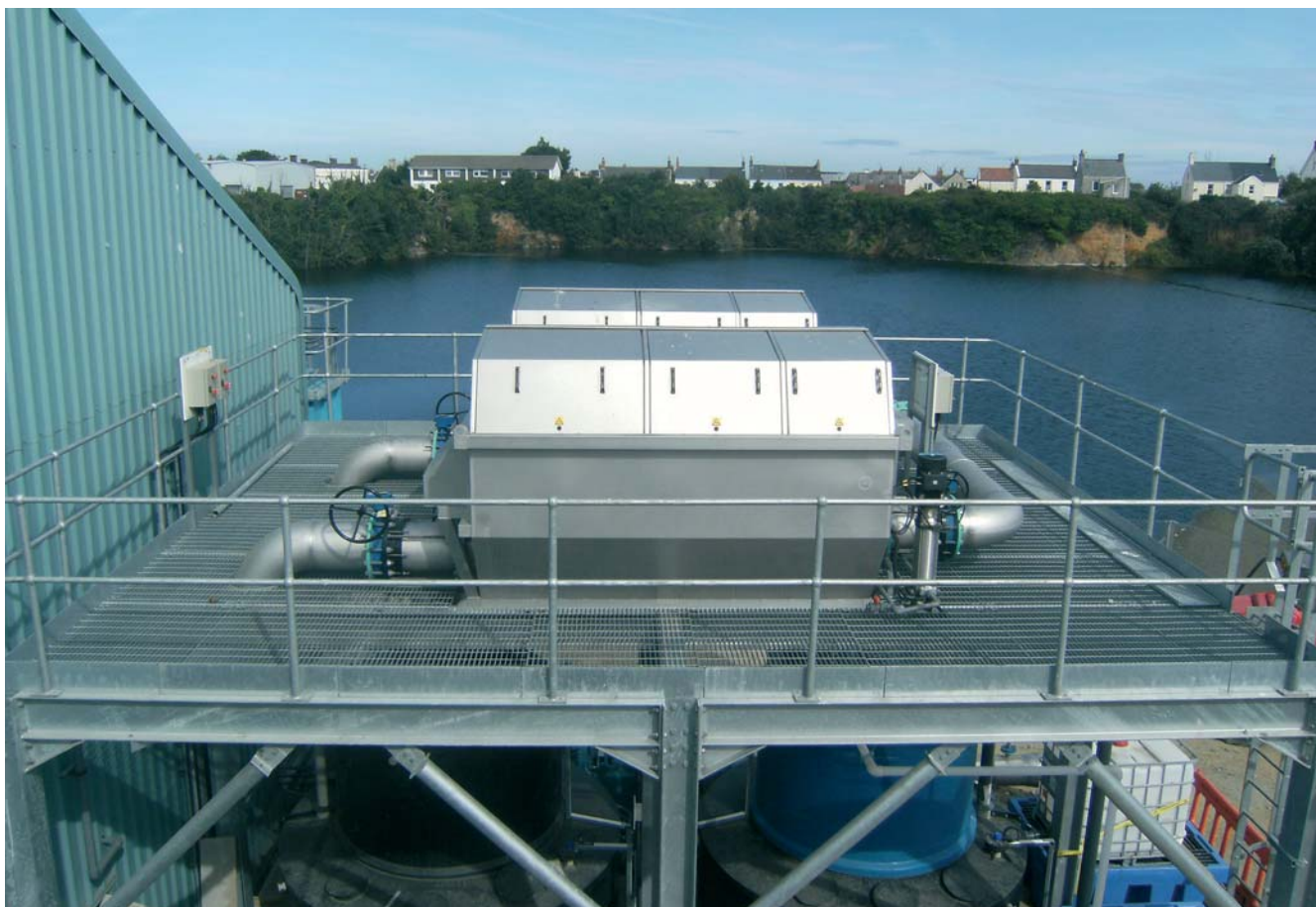
Longue Hougue Microstrainers on inlet of the works
