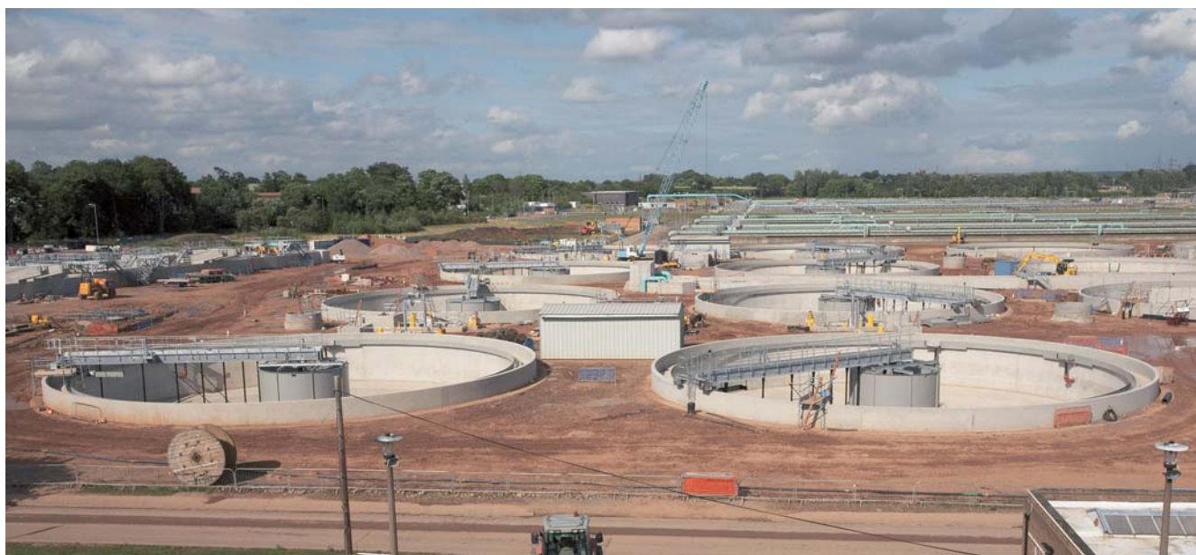
Minworth STW: PST's first batch of 8 bridges installed
