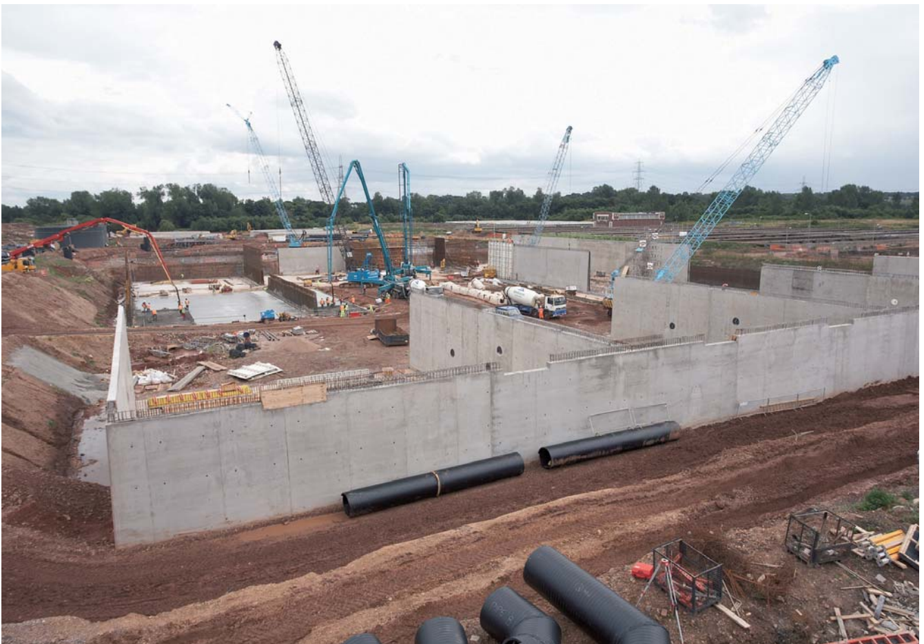
ASP 7 under construction
