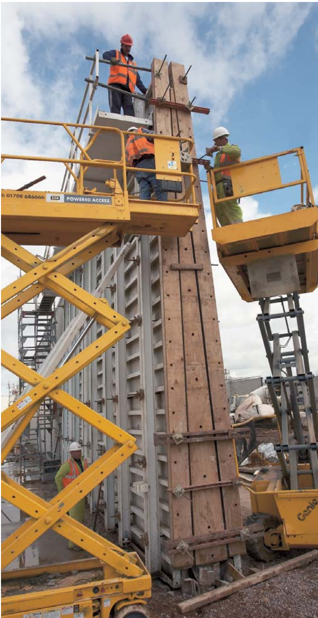
H&S Best Practice - Scissor lift formwork fixing photo courtesy Biwater North Midland Alliance
