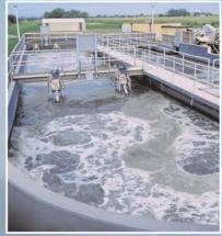
Oxidation Ditch - Activated sludge
