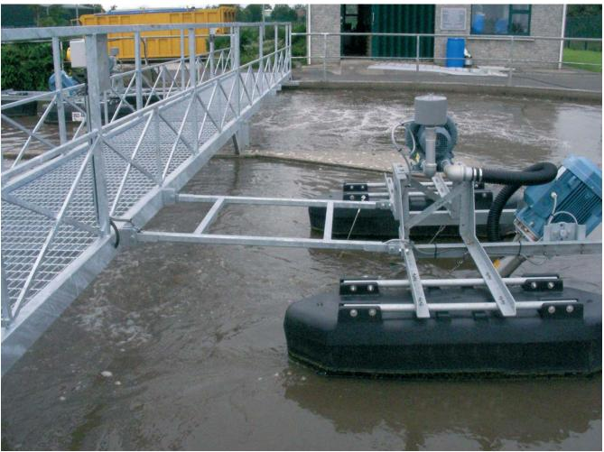
3.7kW Tritons® fixed on a tri-pontoon float. They can be bridge or side wall mounted
