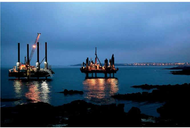
Two large scale rigs were used to lay the 1200m long sea outfall
