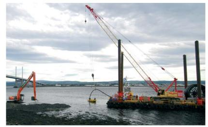
Commercial Marine & Piling installing, trenching and backfilling sewage pumping main across the Beauly Firth in water currents up to 7 knots. 2007
