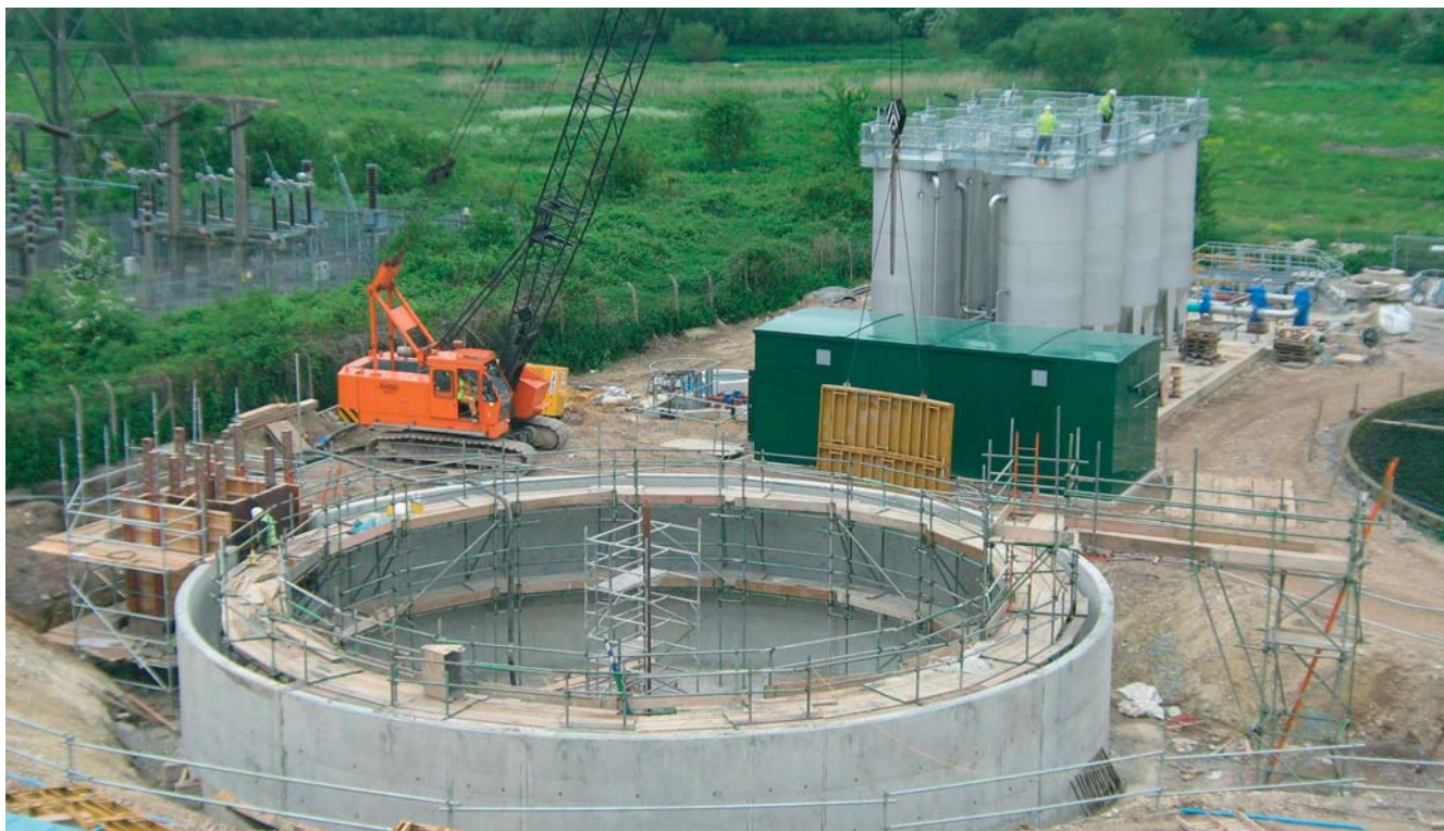
Ratfyn STW under construction
