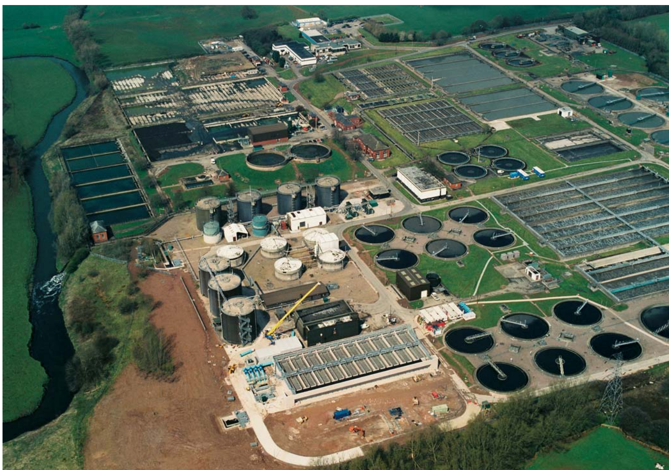
Strongford: The site covers a large area - the NSAF structure to the left of the foreground
