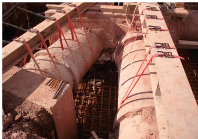
Preparing for work on outfall chamber (left) Preparing overpumping system & Pipes suspended allow outfall modifications courtesy Black & Veatch Europe
