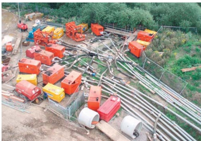
Preparing for work on outfall chamber (left) Preparing overpumping system & Pipes suspended allow outfall modifications courtesy Black & Veatch Europe
