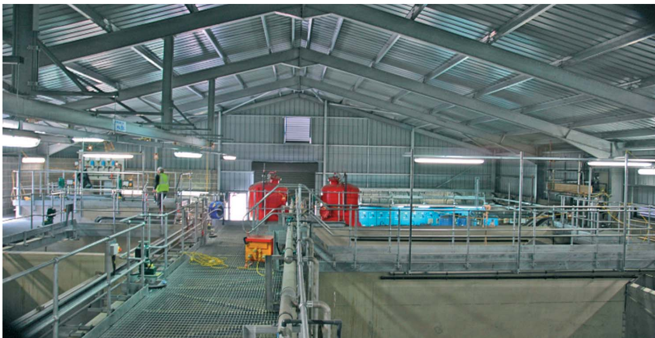
Inside the new DAF building
