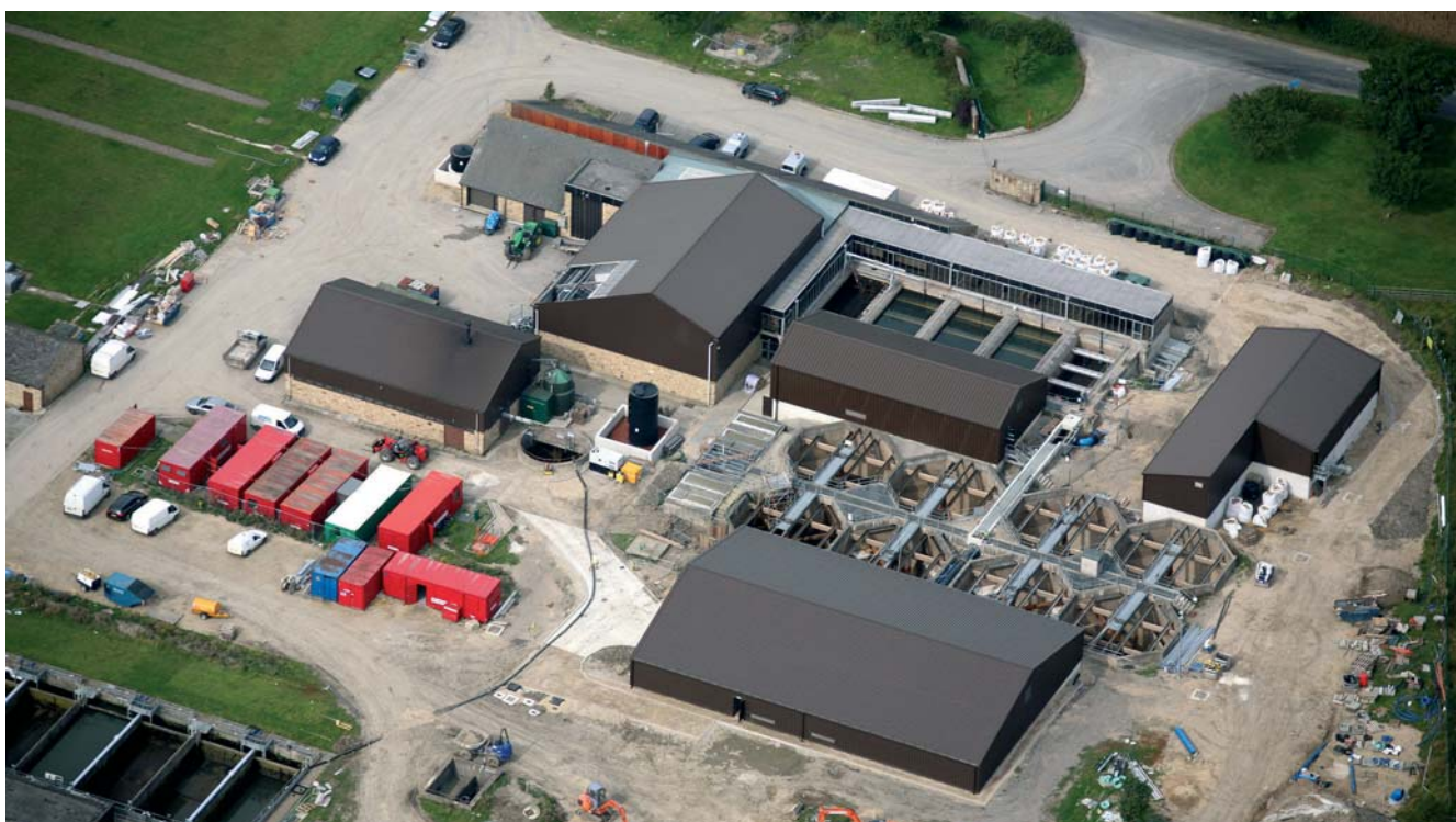
Thornton Steward Works nearing completion
