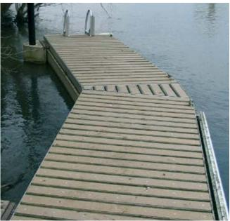
St John's Lock - revenue moorings, new anchorage piles, non slip surface
