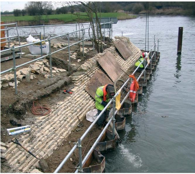
Eynsham - Piles driven and being prepared for timber capping and dry stone wall partially built
