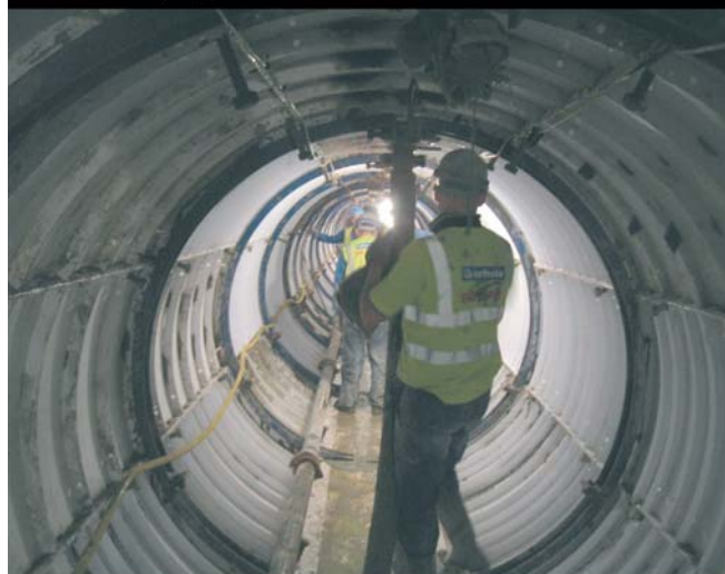
Pumping concrete into the formwork
