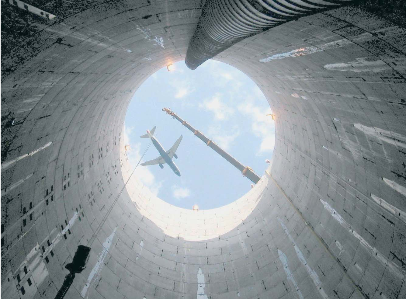
View Skyward from the temporary tunnel access shaft
