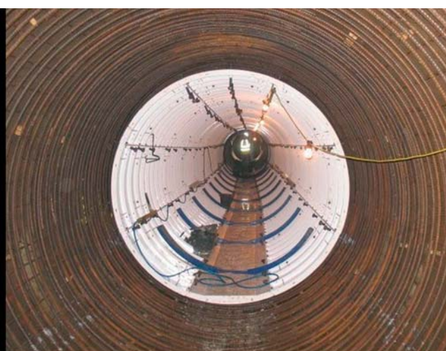
Assembly of the cylindrical formwork
