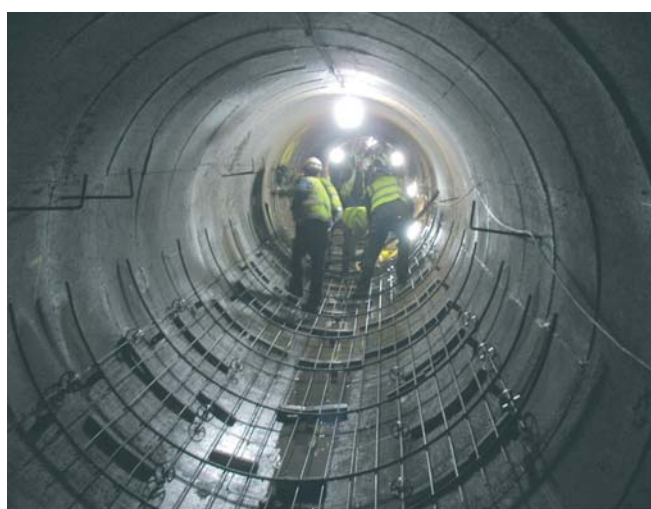
Laying reinforcement within the tunnel
