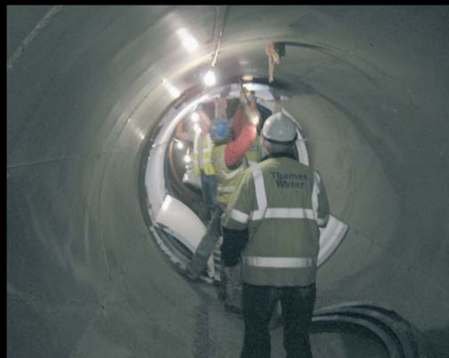
Striking the formwork to expose the finished concrete
