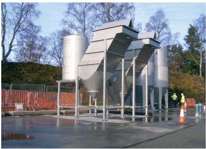
Dynasand filters and Lamella clarifiers before the erection of the new building
