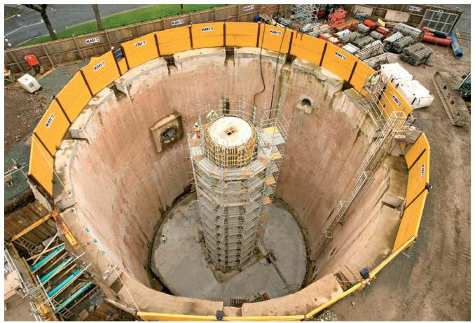
Detention Tank Showing Vacuum Flushing Column Construction
