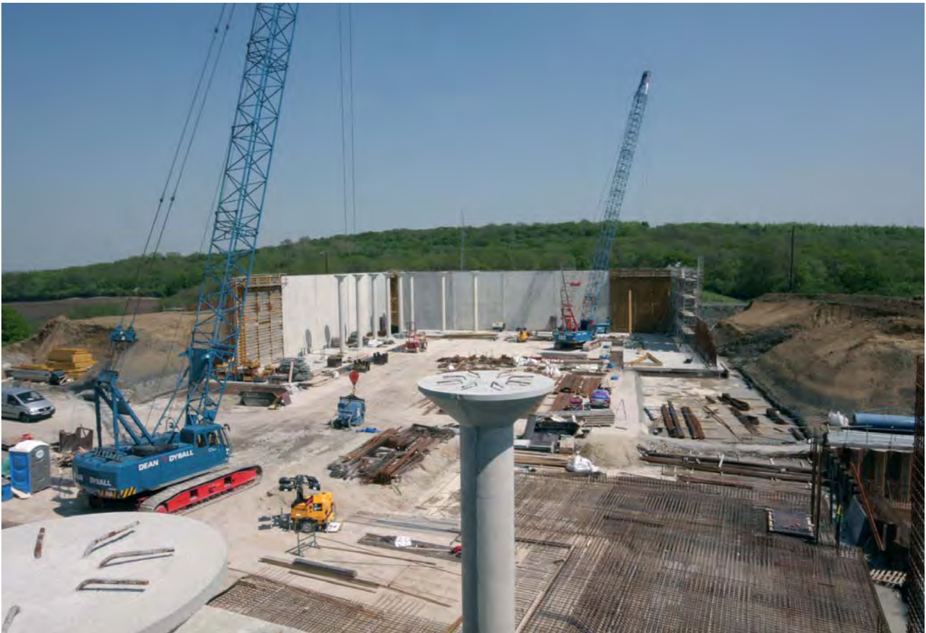
View from outside the reservoirs, during construction
