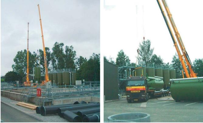
Lifting a new NSF unit into place on the far side of the existing 10 COUF units (left) and offloading 2 new NSF units adjacent to existing 10 COUF units (right)
