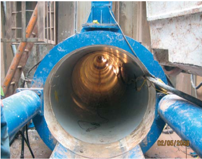
3rd BAFF feed pipe jack in progress (left) and TBM arriving at upstream reception pit (right)
