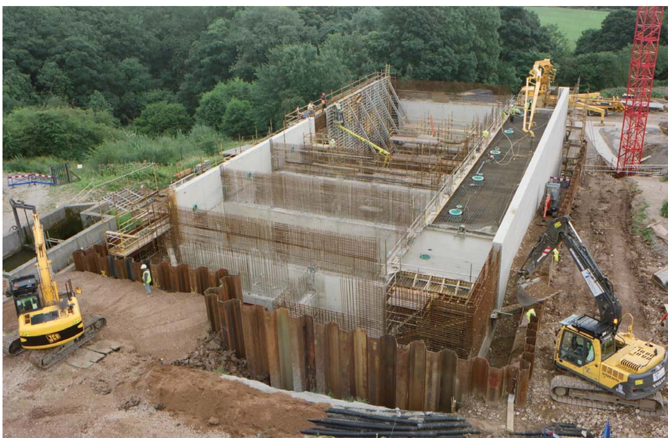
BAFF Structure during construction
