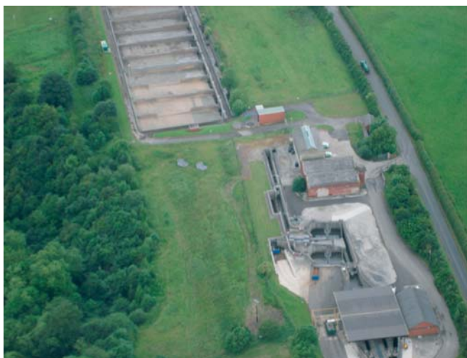
Aerial views of Nab Head Inlet Works (left) and Smithfold STW (right)
