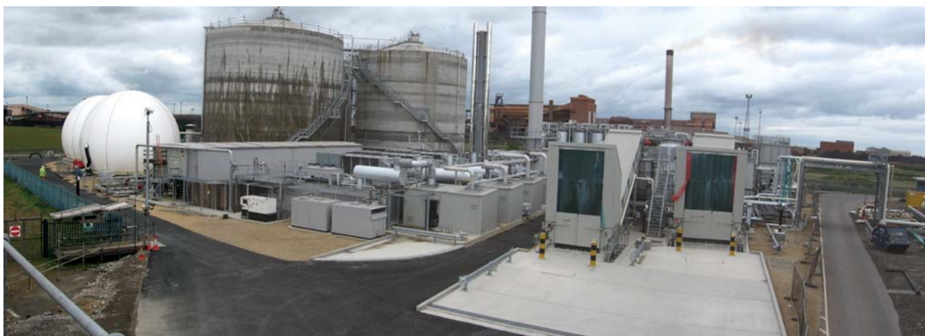
Advanced Digestion panoramic view of site
