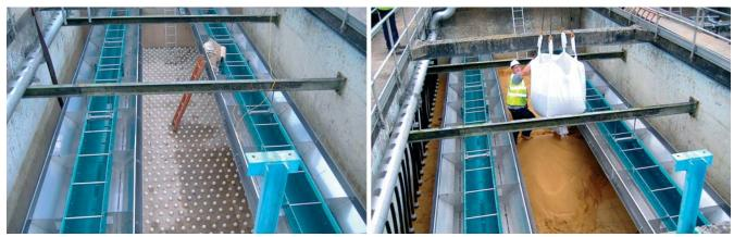
Rapid Gravity Filters. Right photograph shows media being loaded into RGFs
