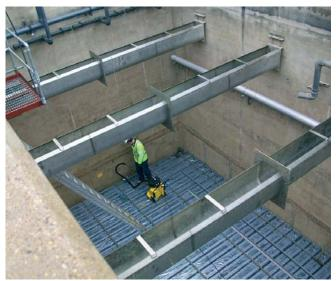
Installation of Leopold Floor in GAC Contactors
