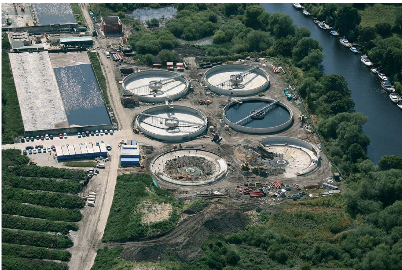
Naburn WwTW - Aerial photograph of the working area
