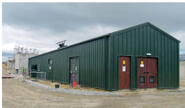
Harrogate WwTW - Electricity substation and welfare building
