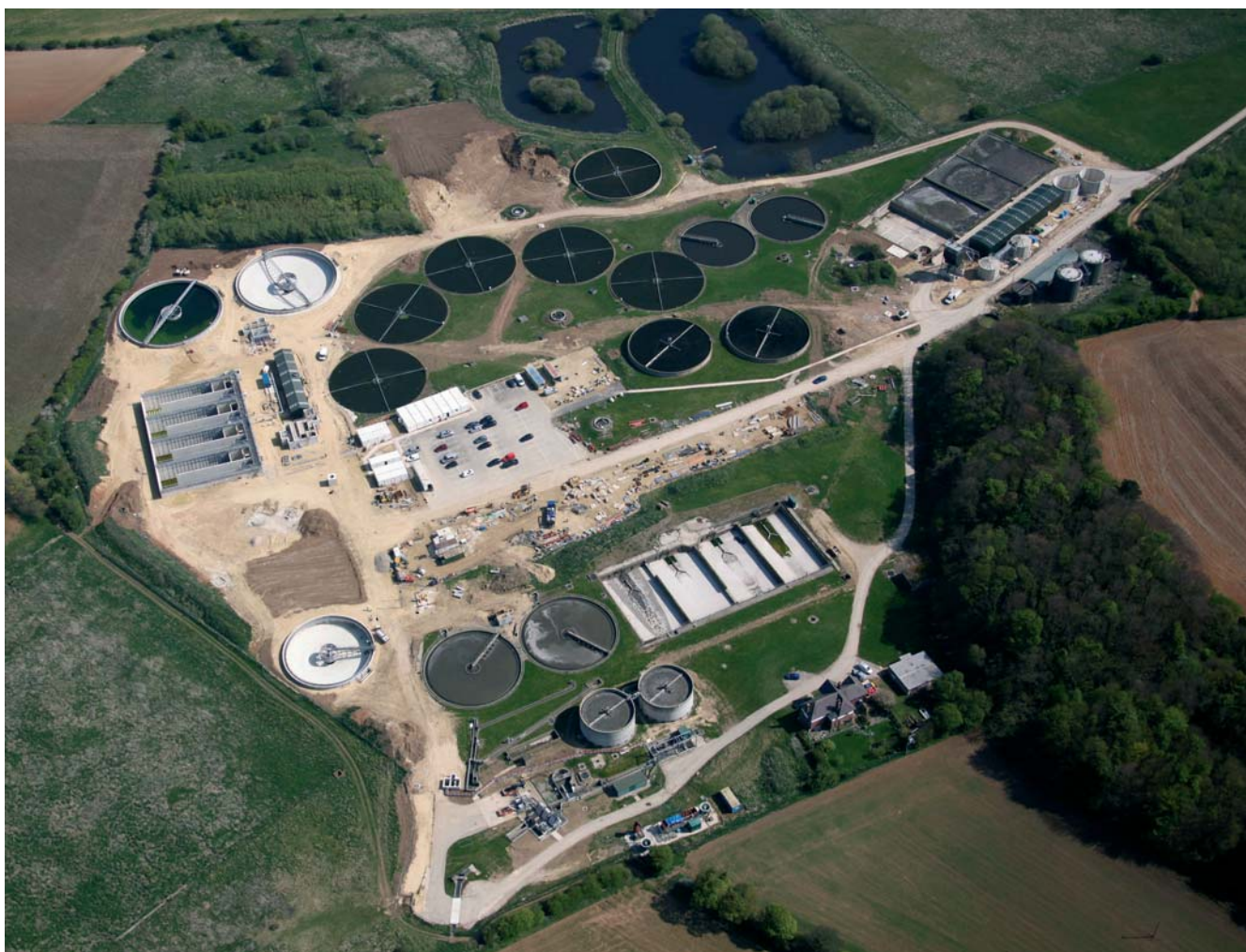
Aerial photograph of Harrogate South WwTW showing construction work
