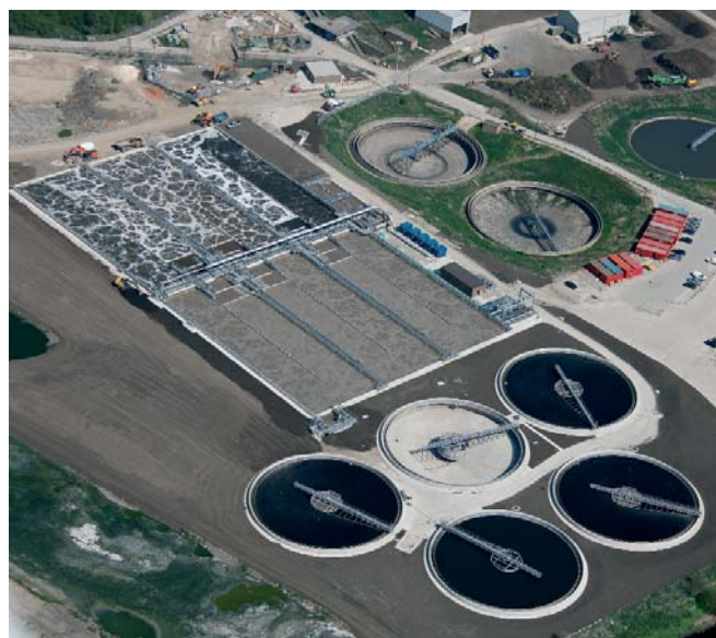
Mitchell Laithes – Activated sludge plant and final settlement tanks nearing completion
