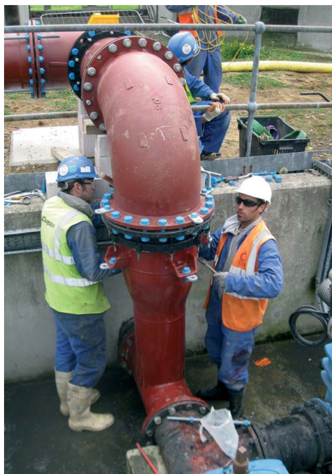
Harrogate WwTW - Upgrading of the pipework at the inlet work
