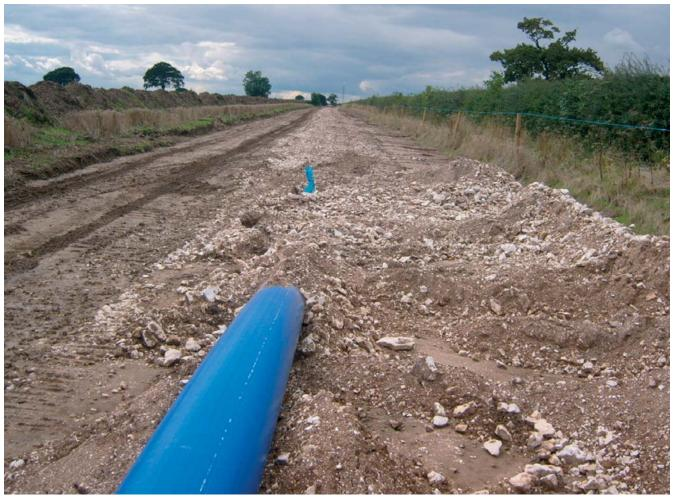
Part of pipeline route now installed by trenching machine
