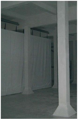
Photograph showing completed works in Tank 1, with sealant coating applied and baffle curtains installed
