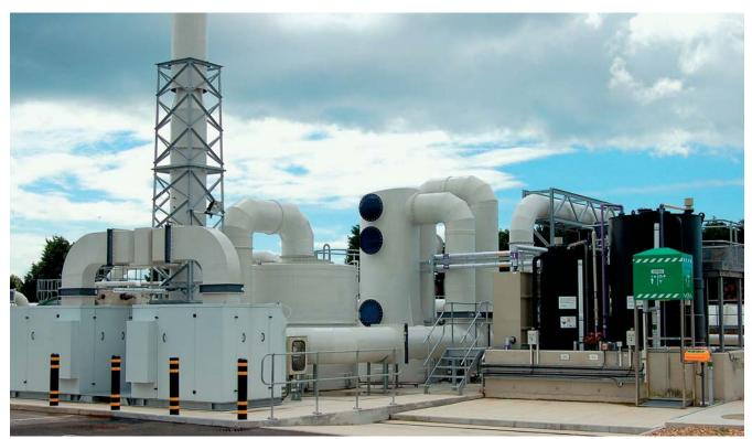
2-stage chemical scrubber system installed in Worthing, a similarly sized plant to that at Kirkcaldy
