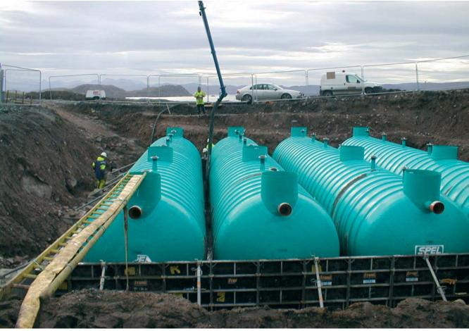
Placing concrete surround to WWTW tanks
