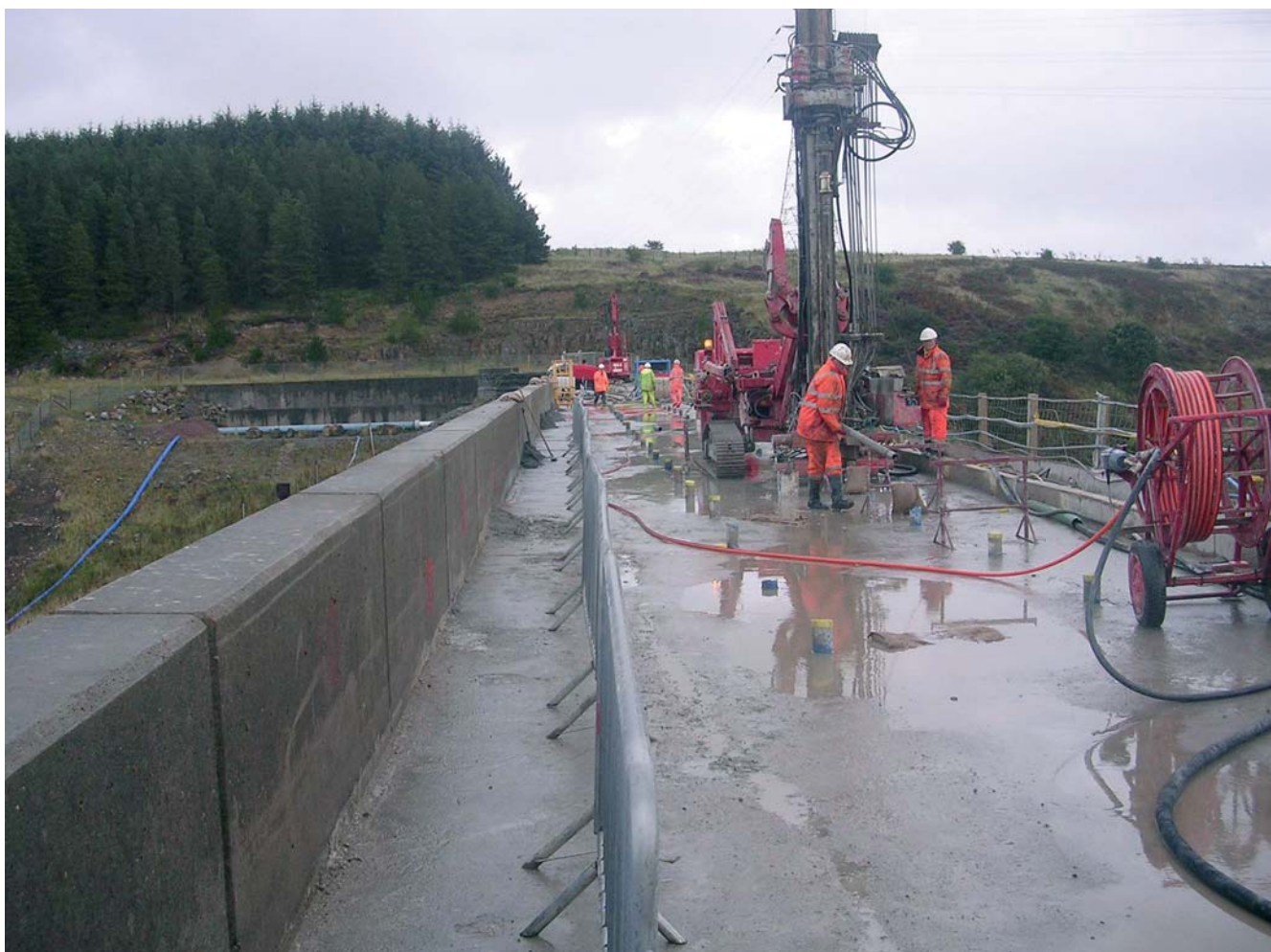
Lower Carno Dam remediation work underway
