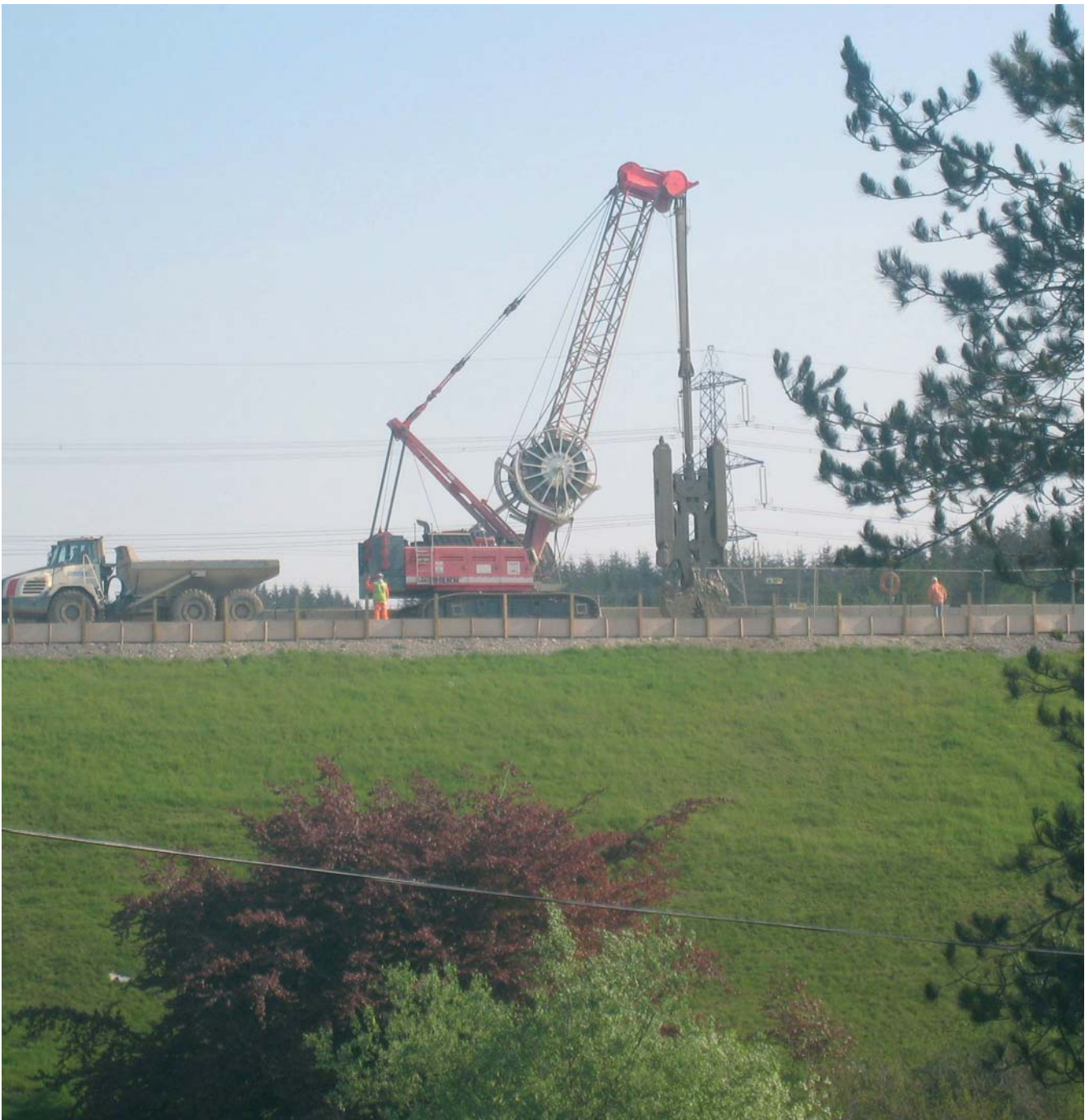
Lower Carno Dam remediation work underway
