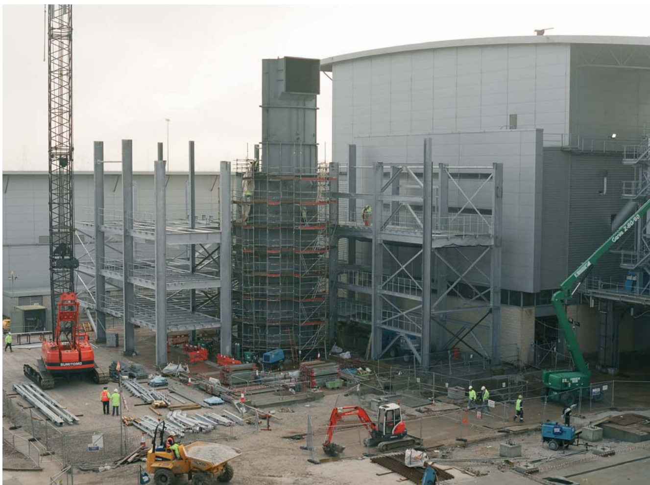
Incinerator construction (January 2009)
