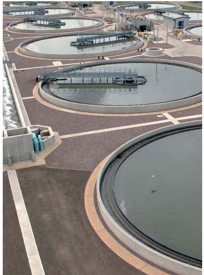
Primary Tank Island and Culverts Courtesy of Biwater North Midland Alliance
