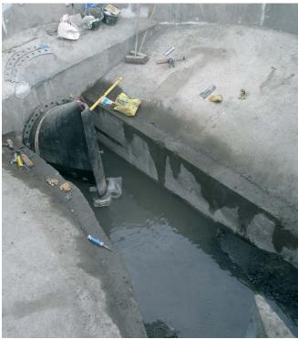
The same Overflow Connection Chamber nearing completion, showing the "Tideflex" non return valve on the 1.05m diameter inlet pipe.
