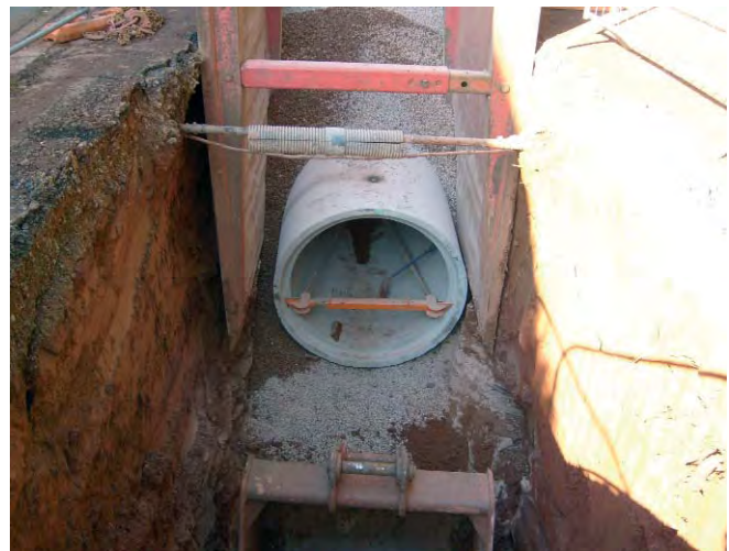
Large diameter storage pipelines under construction
