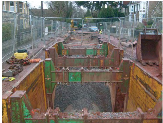
Large diameter storage pipelines under construction
