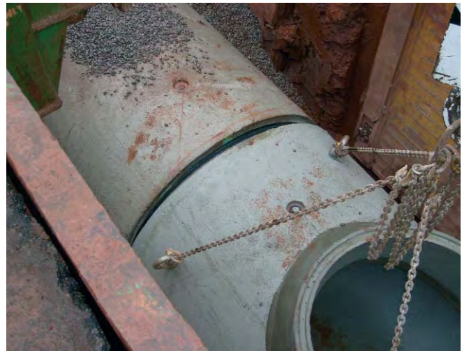
Large diameter storage pipelines under construction
