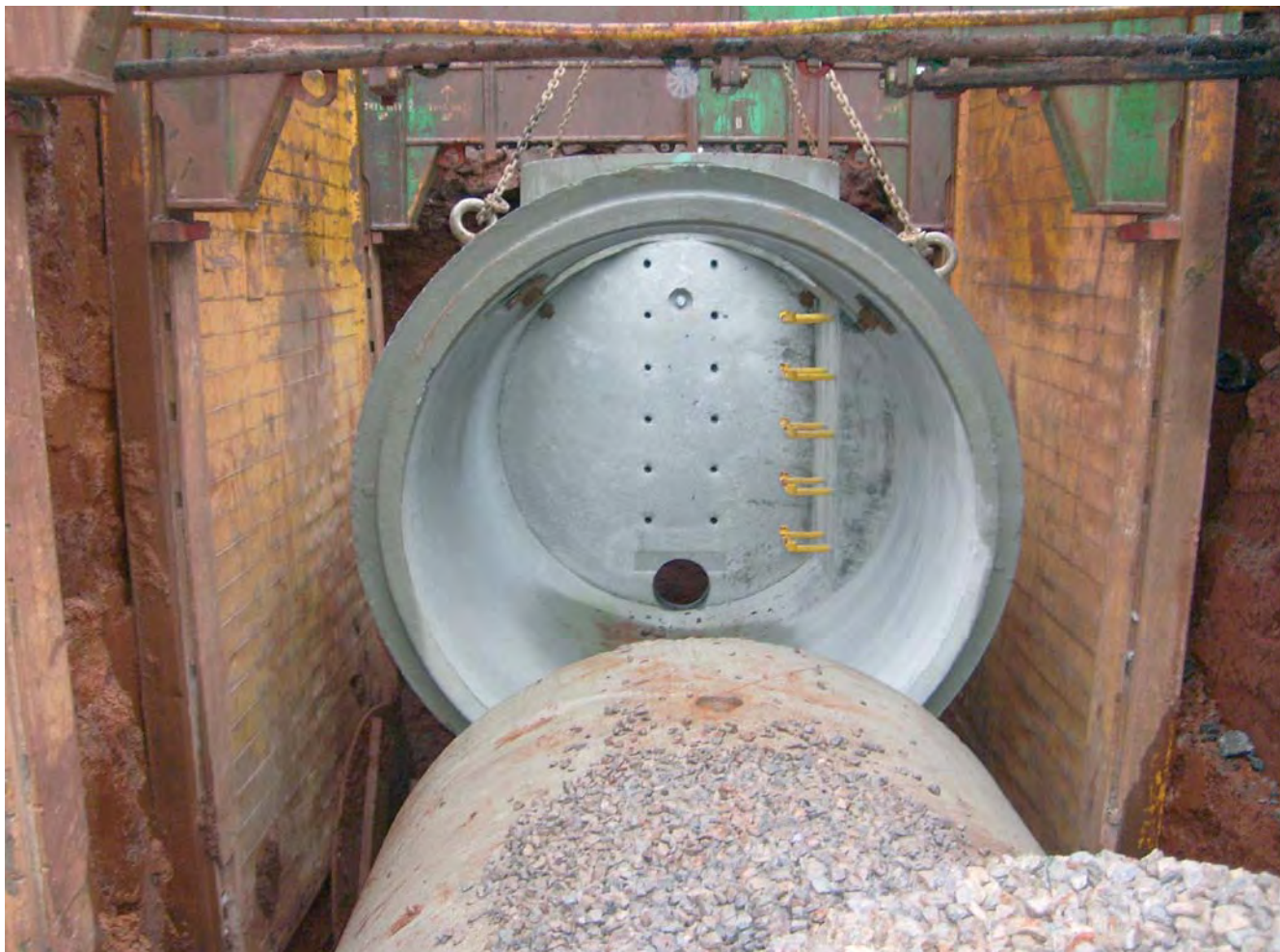
Large diameter storage pipelines under construction
