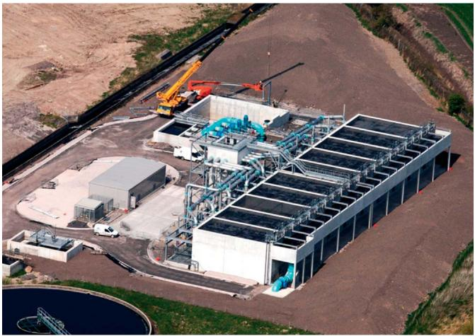
Construction progress March 2009 - pumping station (back left) - MCC Kiosk (front left) BAFF Plant and Distribution Chamber (right)
