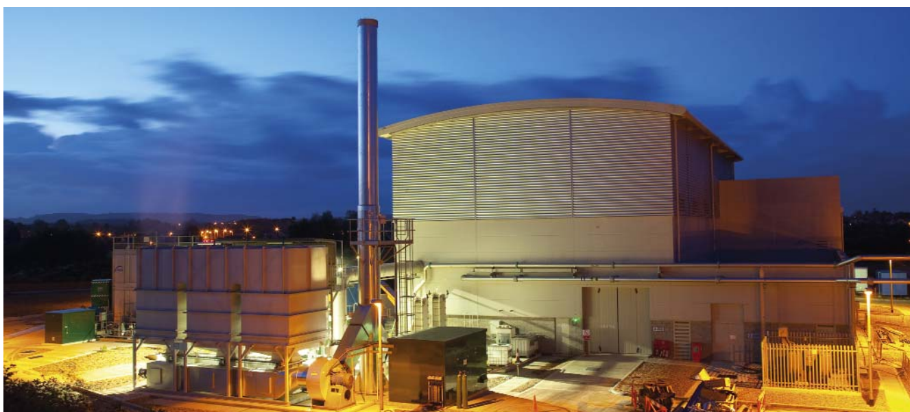
Ashford Sludge Treatment Centre
