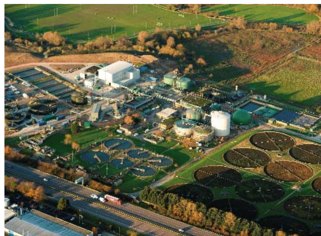
Aerial photograph of Ashford WTW and STC
