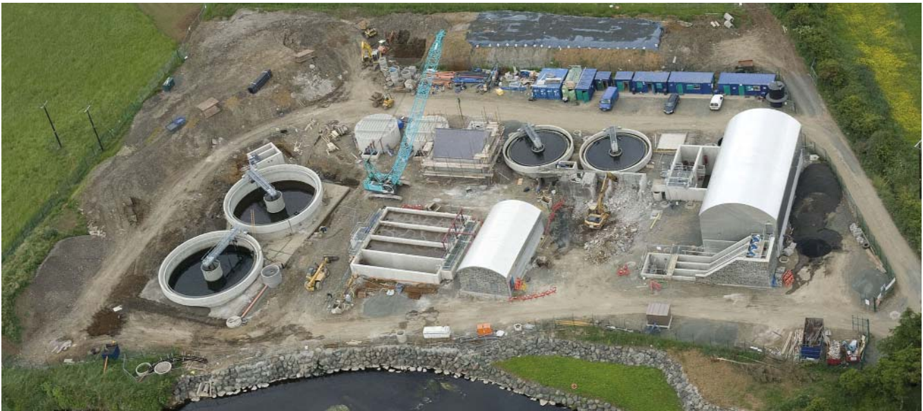
Aerial photo of Bushmills WwTW June 2010
