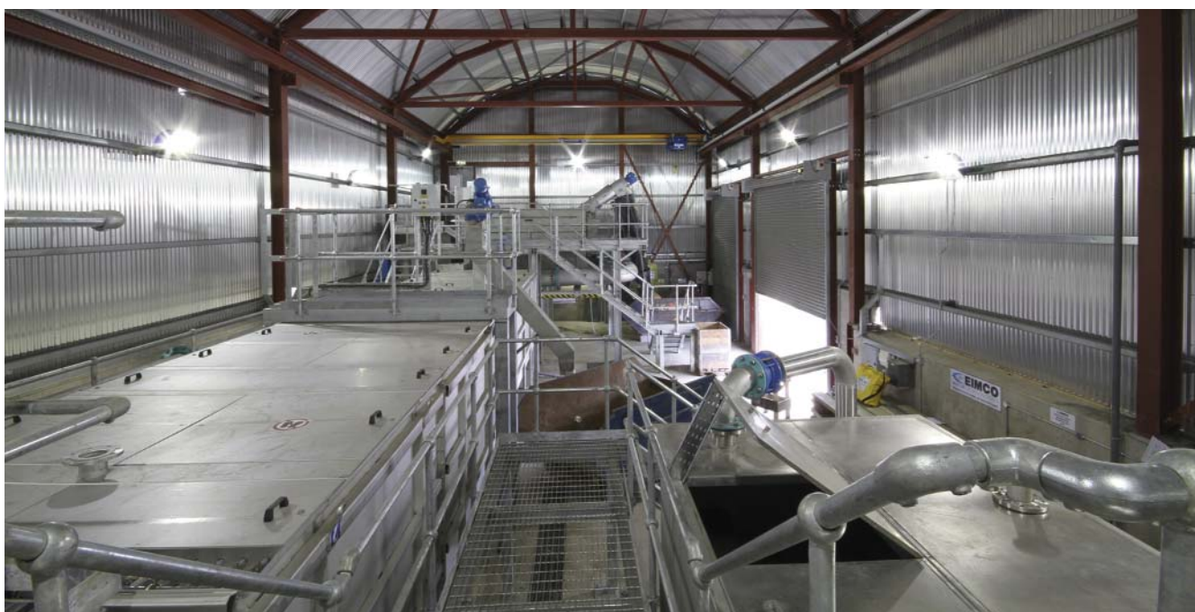
Inside the inlet building May 2010
