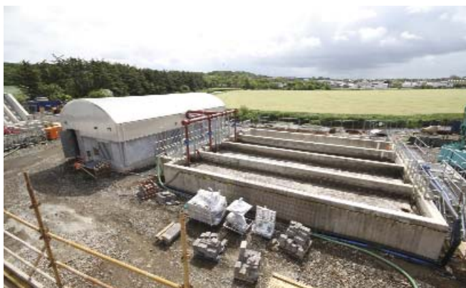
Bushmills WwTW - MMC building and aeration lanes May 2010
