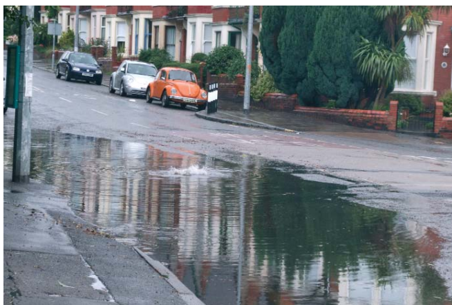
Flooding caused by overflowing sewer network in Cardiff East
