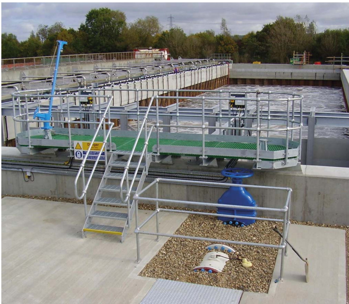
Aeration lane and anoxic zone view
