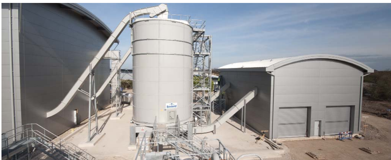
From left to right: sludge treatment building, sludge cake silos, truck loading tunnel
