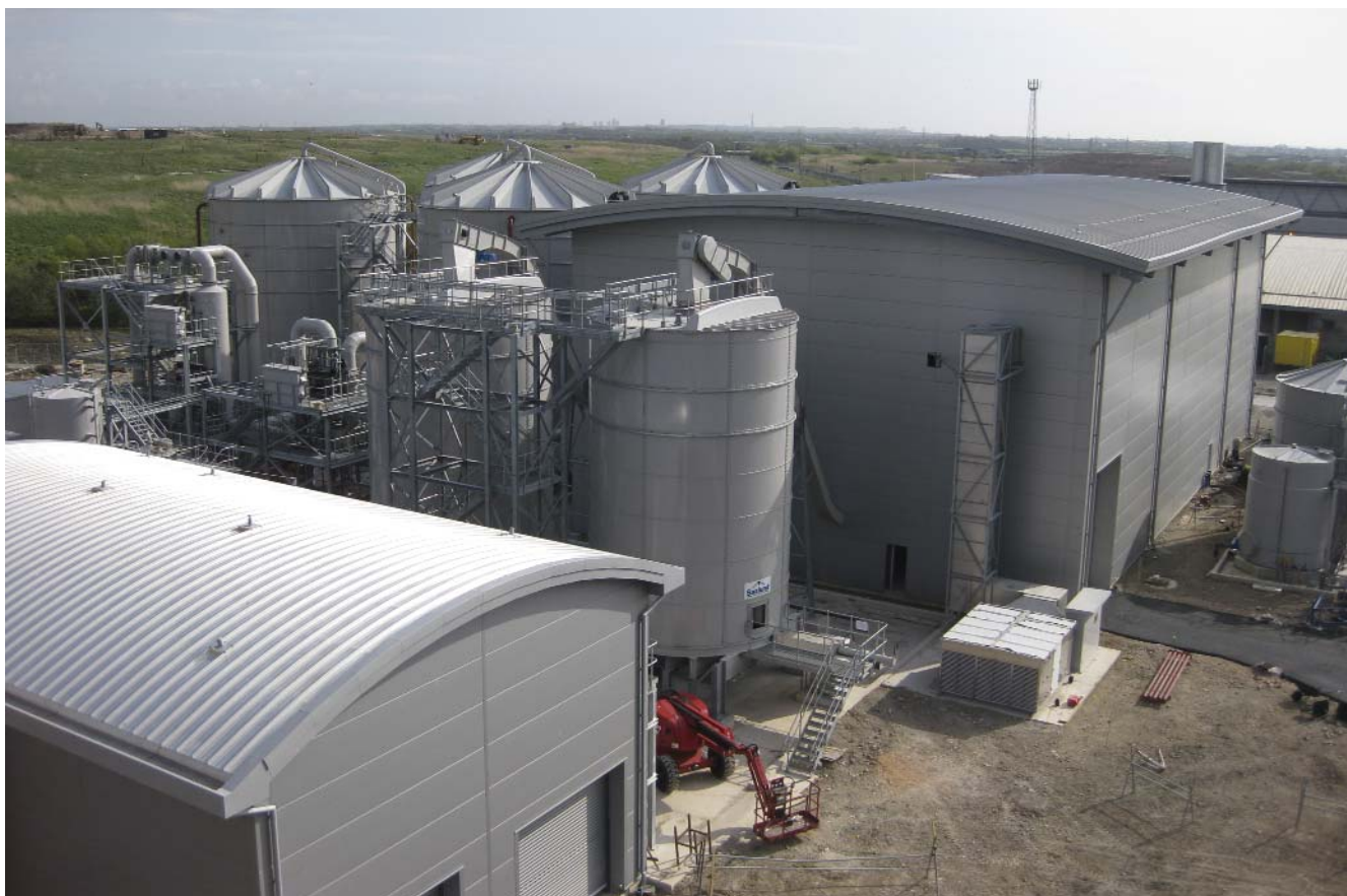
From back to front: sludge storage tanks, treatment building, odour control plant, cake silos and truck loading tunnel
