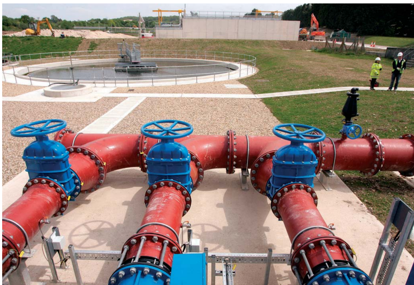
Fullerton Wastewater Treatment Works
