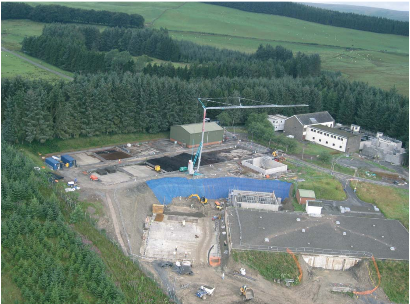
Aerial view of Robertson WTW Construction Phase
