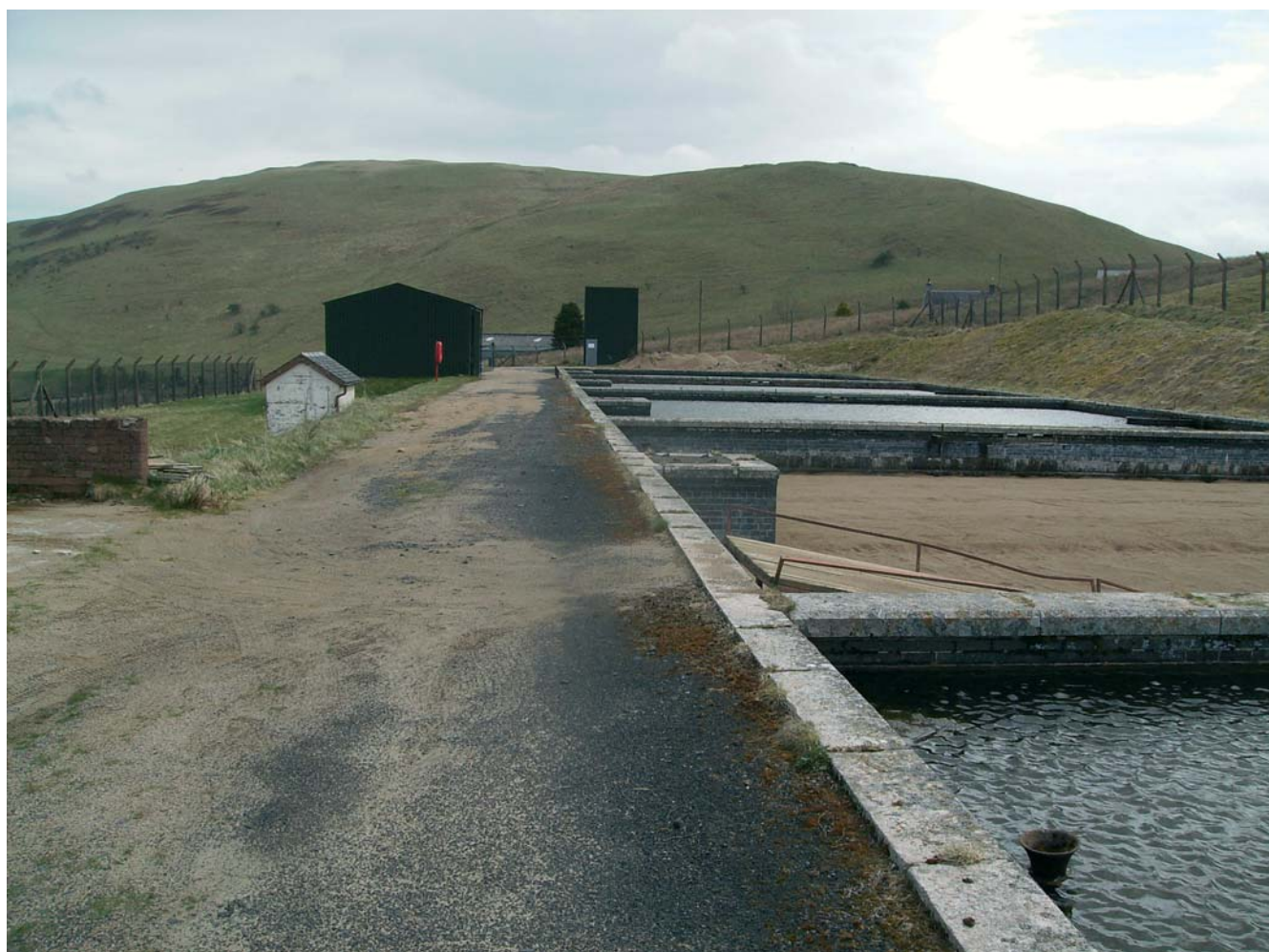
Dodburn WTW – Existing works to be abandoned included slow sand filtration beds and disinfection processes
