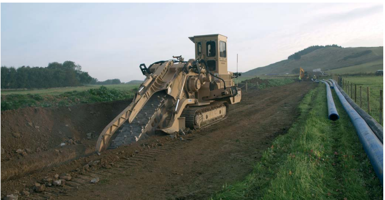
Trencher excavating for rising main
