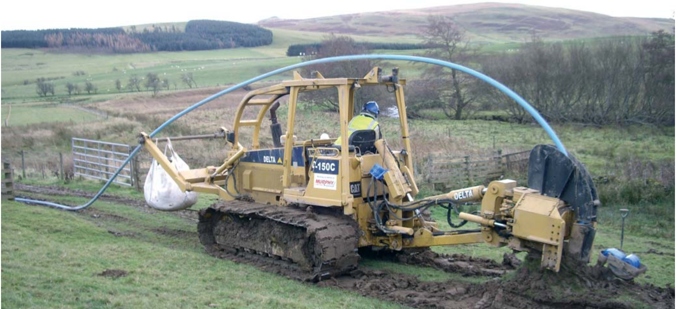
Mole Plough installing alkothene pipe across fields
