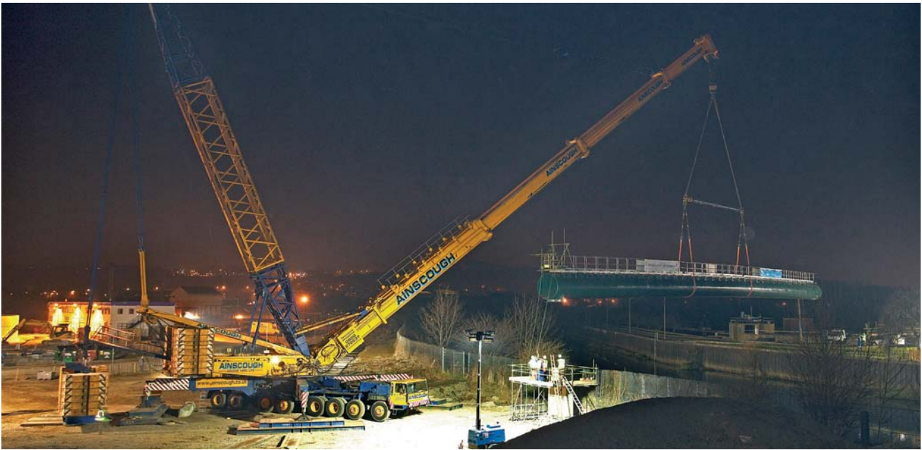
Lifting the pipebridge into position
