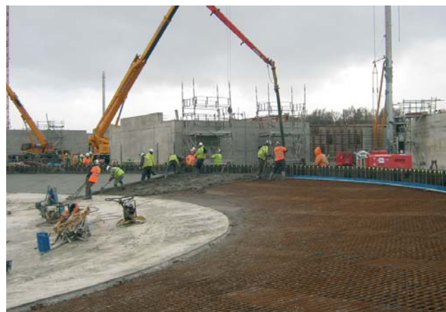
Final Settlement Tanks Construction
