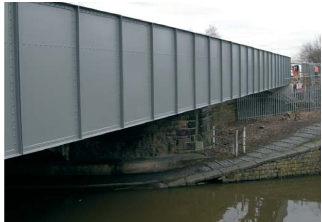
Dewsbury Cut Pipebridge
