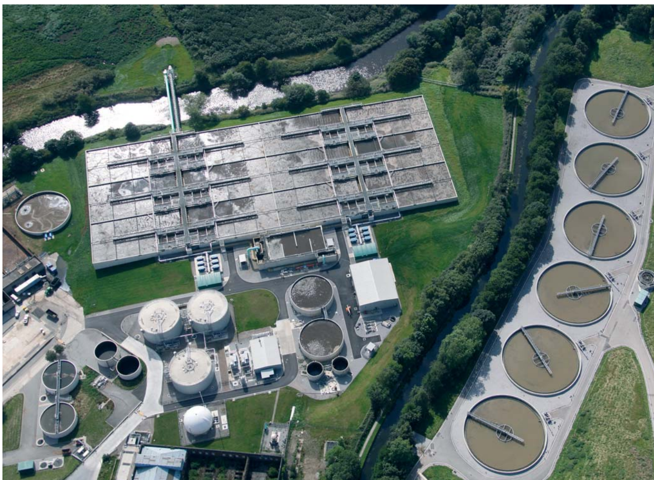
Esholt WwTW: Activated sludge plant to left (part of Phase 2) and primary settlement tanks to right (part of Phase 1)
