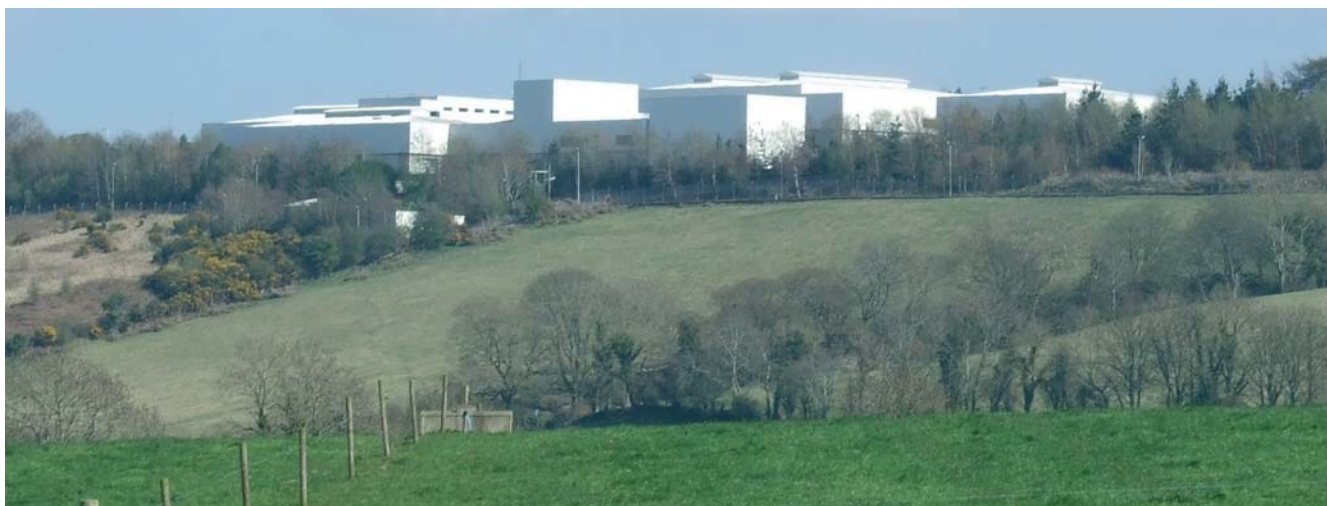
Carmoney Water Treatment Works
