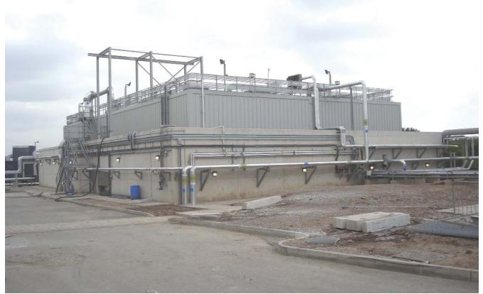
General view of completed plant within concrete bund to meet IPPC requirements (May 2010)
