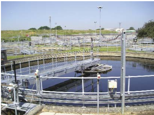
New Scraper Bridge installed in existing Final Settlement Tanks
