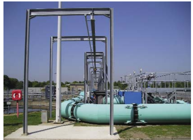
Pumping station 4A and Overhead Gantry
