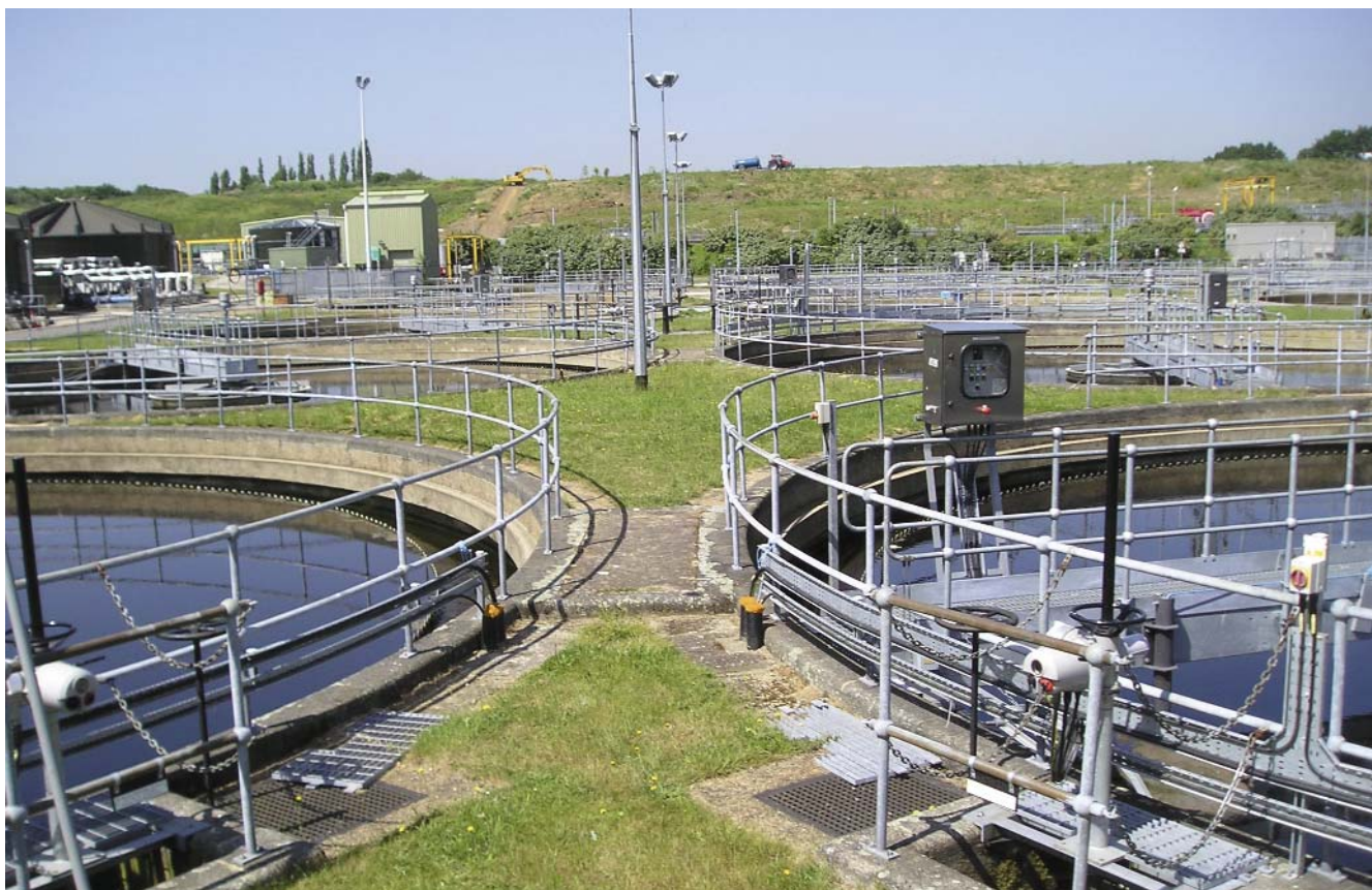
View across Final Settlement Tanks
