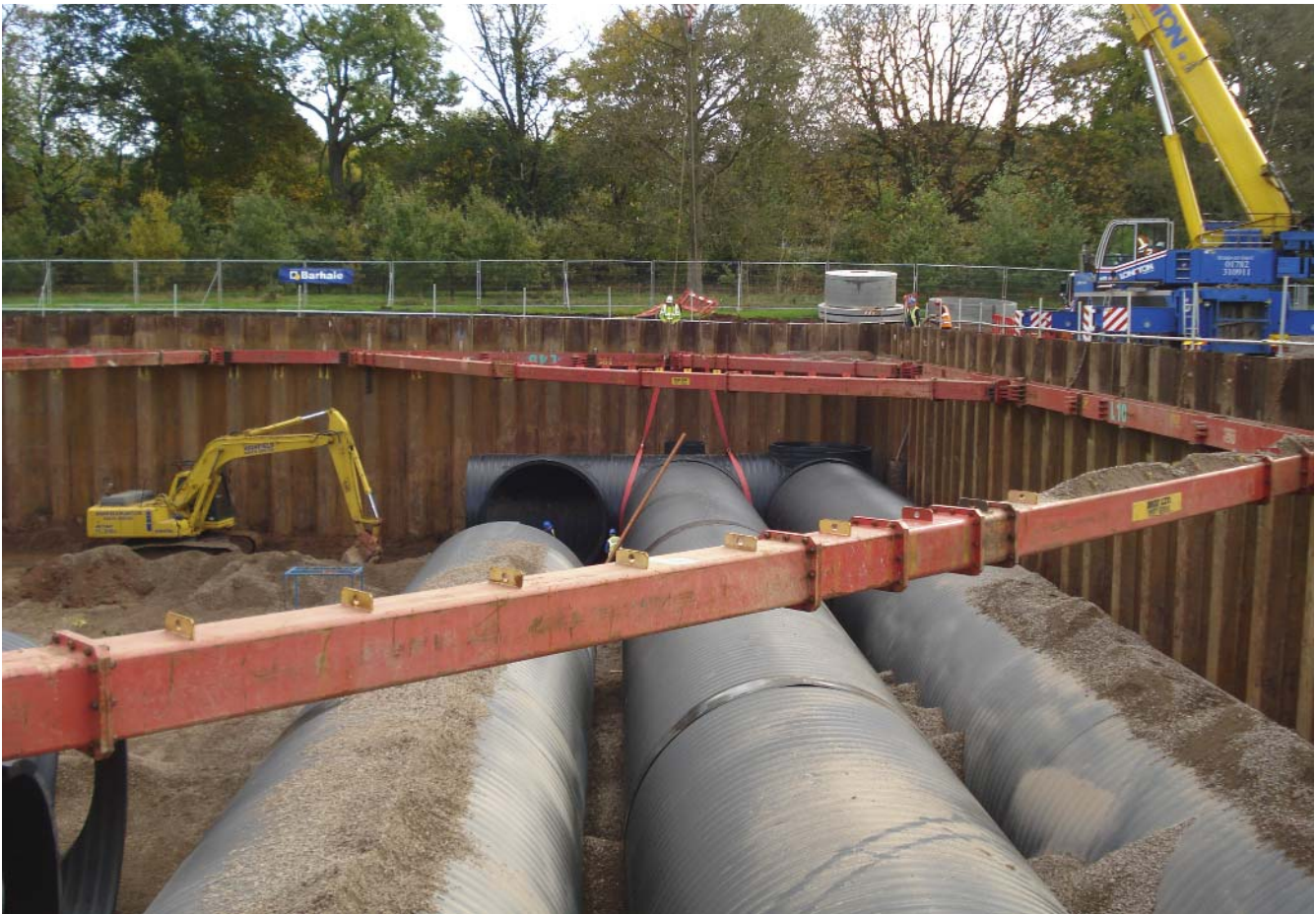
Weholite tank construction
