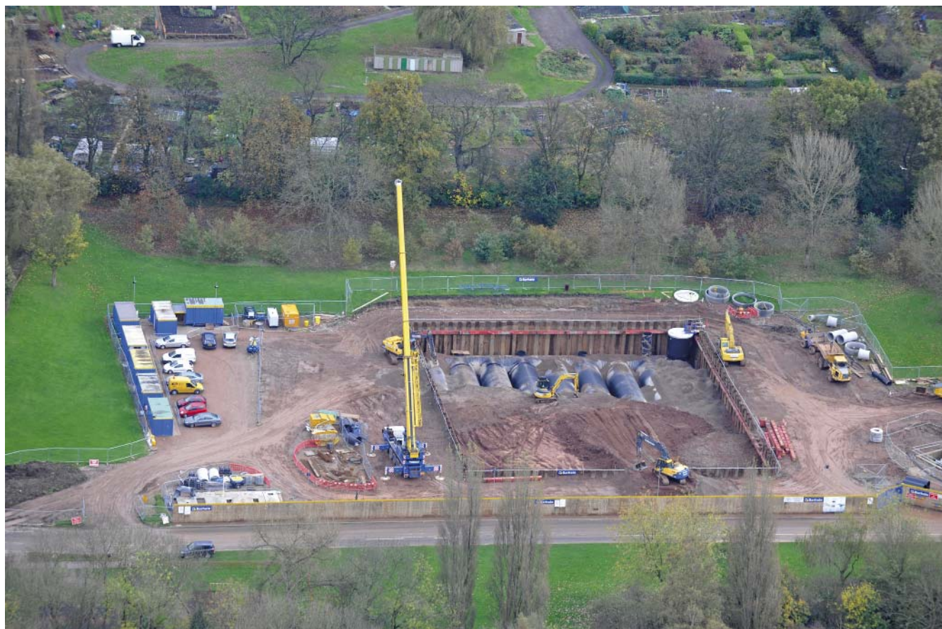
Aerial View of storage tank site
