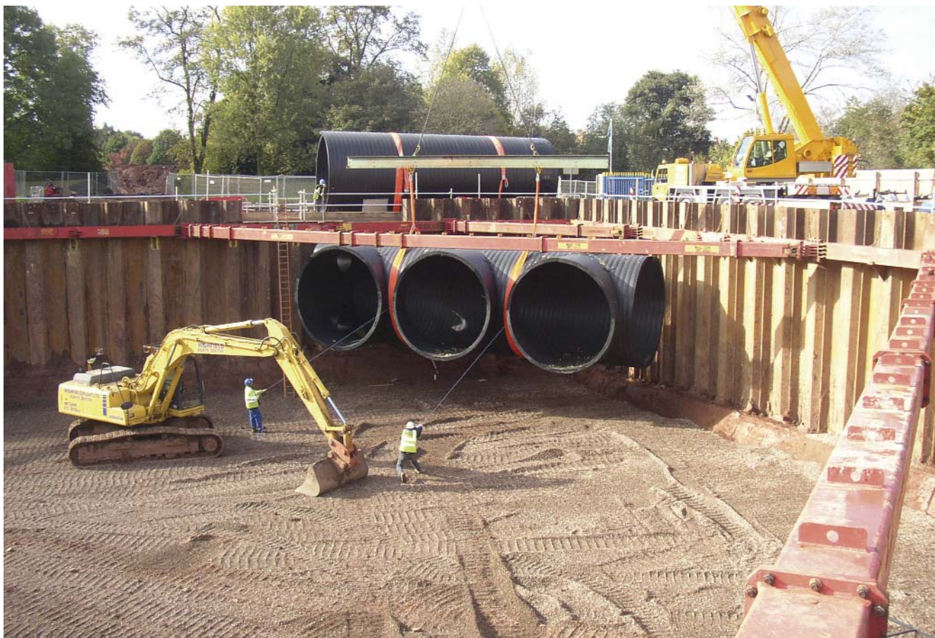
First Weholite manifold placement
