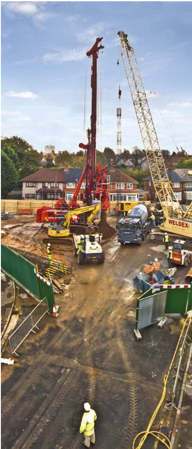
Foxton Road Site during piling works
