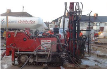
Drilling of Jet Grouted Columns
