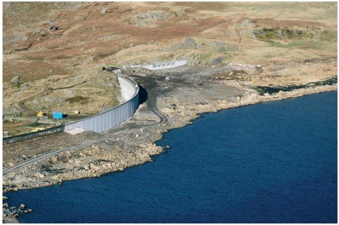
Aerial view, upstream face of concrete dam and auxiliary overflow showing temporary access and Carpi Membrane Courtesy of Eric Wright Civil Engineering Ltd and MWH
