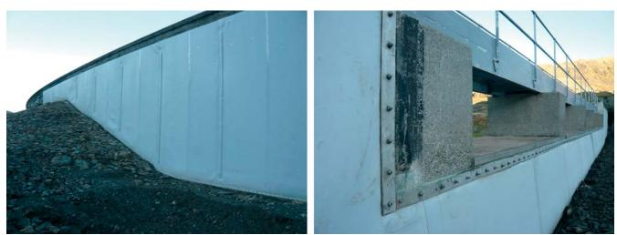
Photos show new membrane on upstream face of concrete dam (left) and auxiliary overflow (right)
