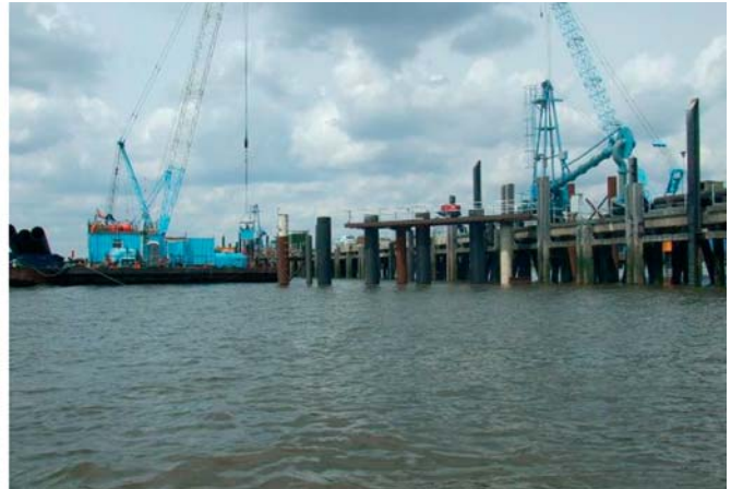
View from River Thames during construction of the extraction platform
