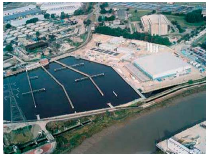
Aerial view of buffer tanks
