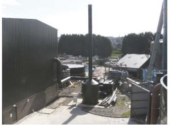
Odour Control Plant (Carbon Filter, Stack, Biofilter and Ducting)
