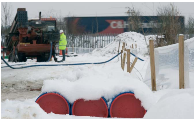
Directional drilling under M20 during the snow
