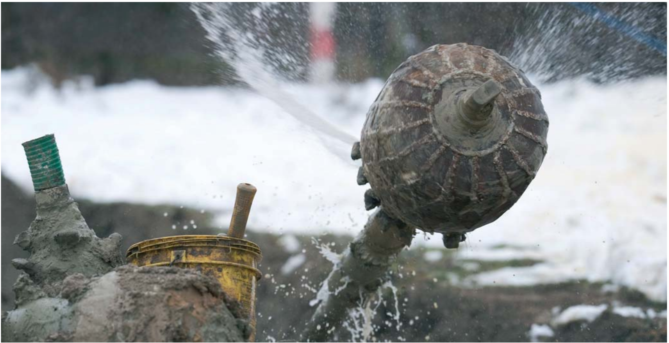
Contact and backwash tanks during construction
