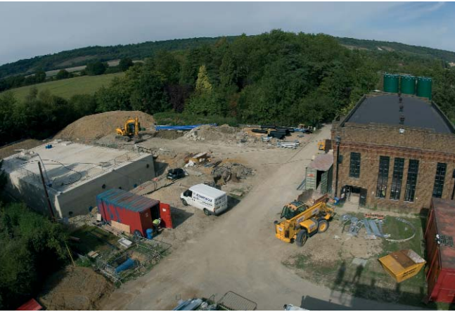
Construction site Photograph by Ady Kerry, courtesy of South East Water
