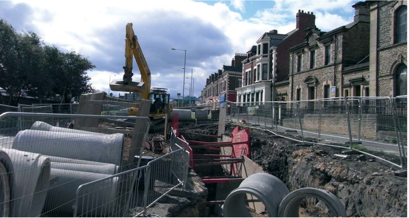
Restricted working area at High West Street in Gateshead
