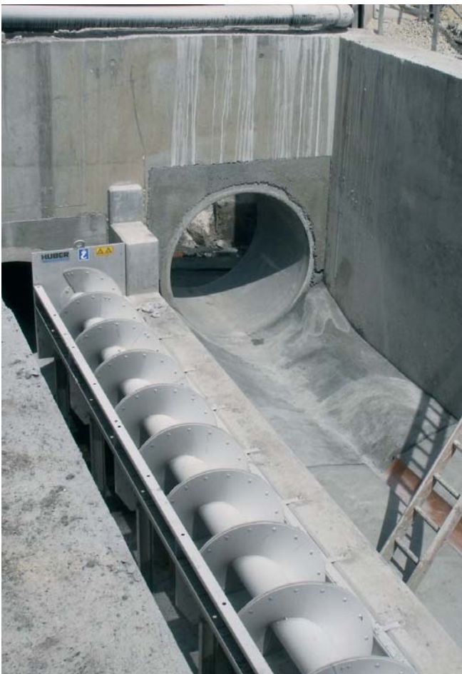
(Left) Huber ROK1 mechanical screen at new build Eldon Street CSO, and (right) Huber ROK2 mechanical screen retrofit into the Rose Street
